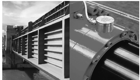
Figure 7. CIMS integrated in cylinder of preventing tides control system in Saigon river
