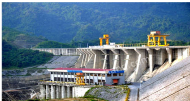
Figure 1. Hydroelectric power plant
