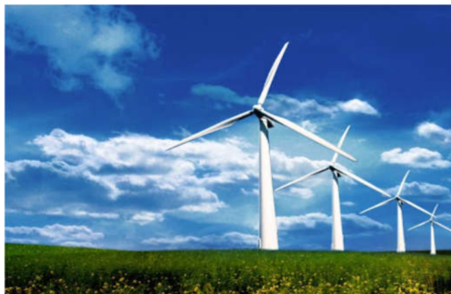
Figure 4. Wind power plant
